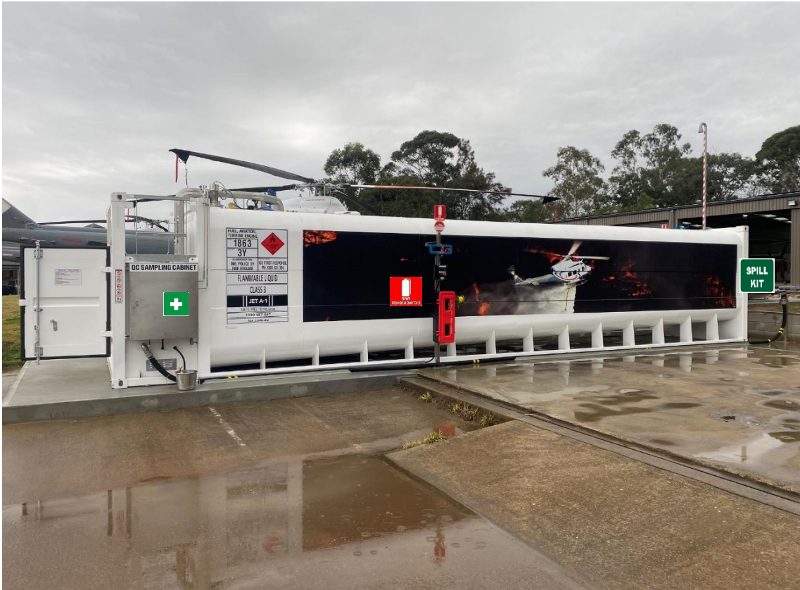
Refuelling bowser with fire extinguishers and spill kit
