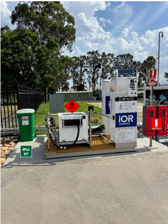
Refuelling bowser with fire extinguishers and spill kit
